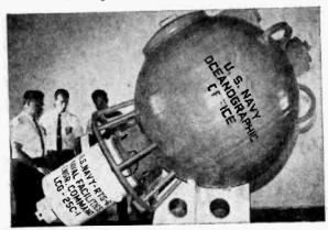
Undersea radioisotope generator by Martin Marietta will power oceanographic buoy for beaming data to ships and planes.
